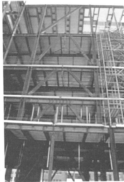
b. Split-K-braced frames
